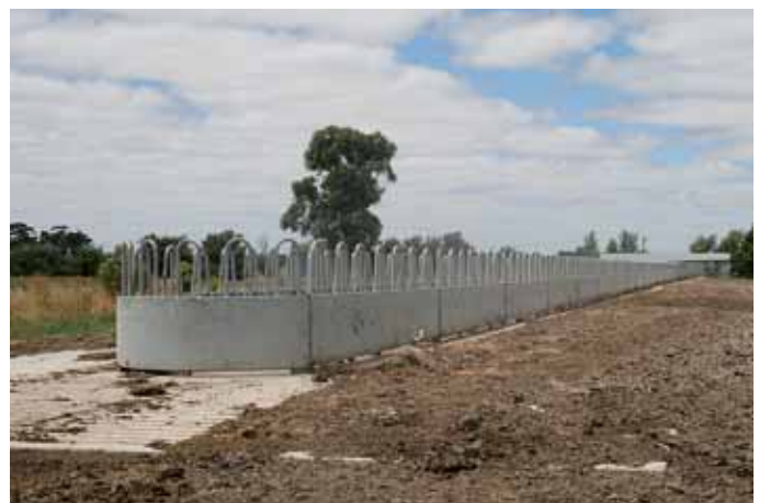
Figure 7.2 – Concrete Feedpad with modular steel troughs, combined feed and drive alleys
