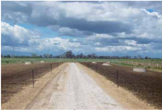
Figure 1.1 – Semi-permanent Feedpad with rubble drive alley and 2 hot wires
