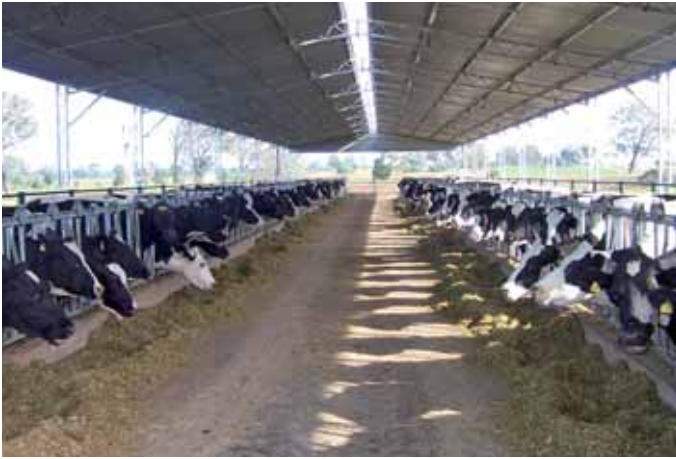
Figure 7.3 – Covered Concrete Feedpad with central drive alley, 2 feed alleys and stanchions
