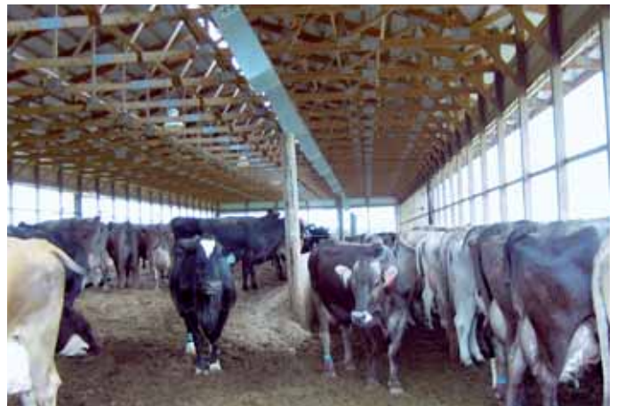
Figure 7.6 – Covered Compost Barn with sawdust bedding (raised bedding area on the left; feed alley on the right)
