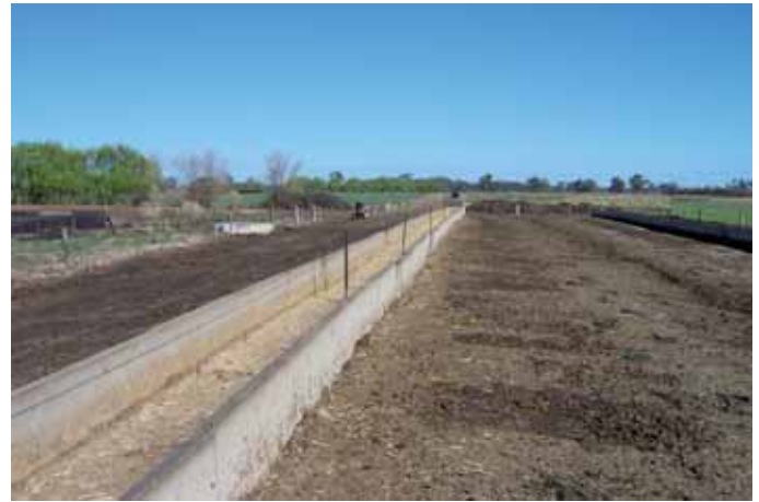
Figure 1.2 – Semi-permanent Feedpad with concrete modular troughs and a central hot wire
