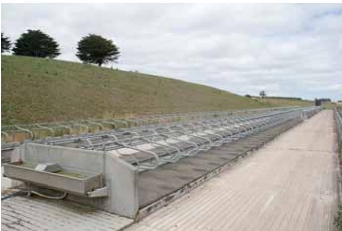
Figure 7.5 – 6-Row Uncovered Freestall with rubber matting, central drive alley, 2 feed alleys and 2 cow alleys
